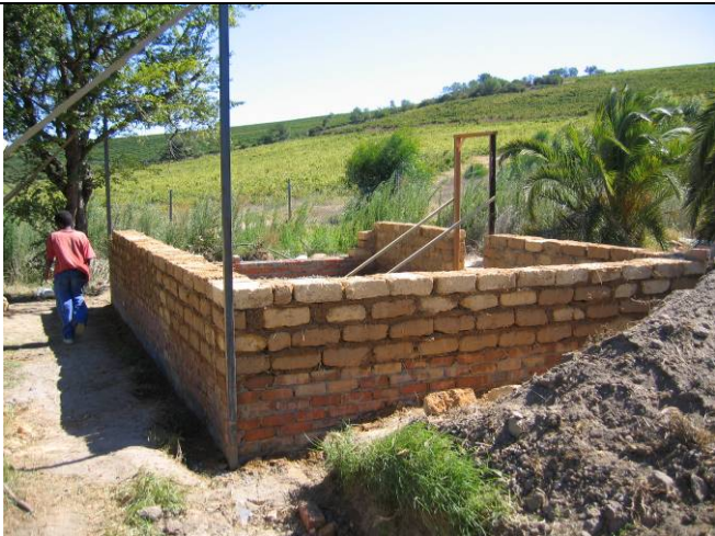
Figure 4: View showing conventional brick and adobe layers
