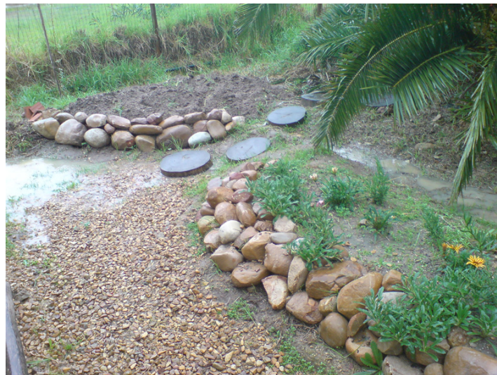
Drainage through simple swales
