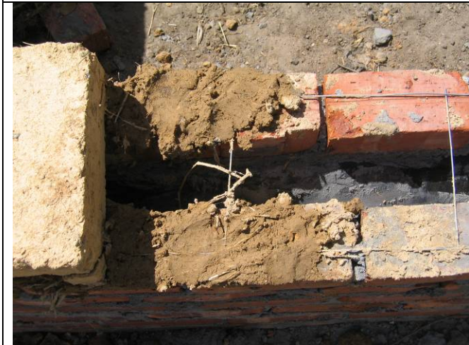
Figure 3: Interface between conventional clay brick and adobe
