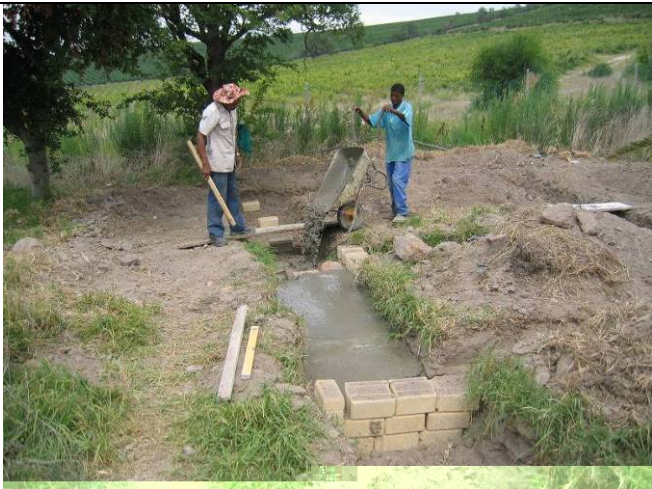
Figure 2: The conventional concrete foundations
